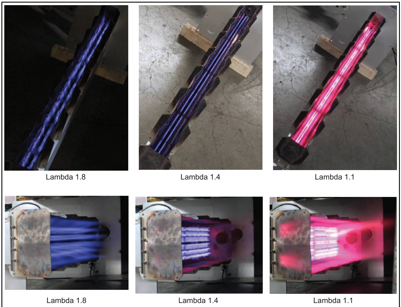
Figure 4.3. Low Fire Flame Appearance
